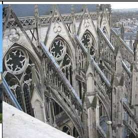
Fig.3: Flying buttresses of Amiens Cathedral 1270 (5)
