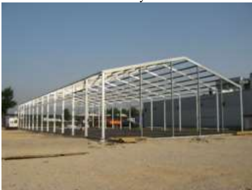
Figure 14: Shows the steel structure warehouse
